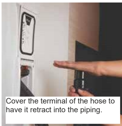
Closing the cover you switch off the unit.
